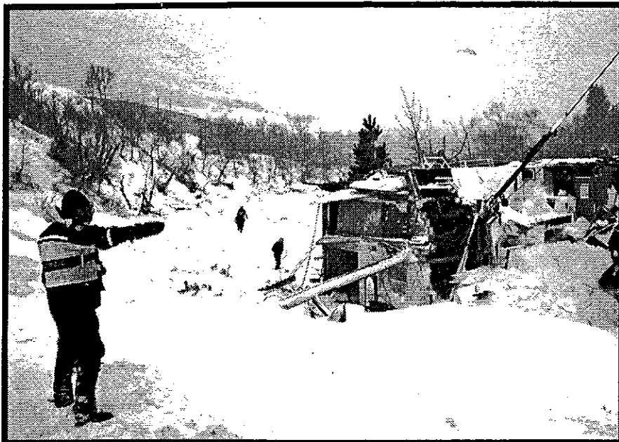
The historic and spectacular January slide cycle caused damage to the bottom terminal of the Bridal Veil Falls tram.
